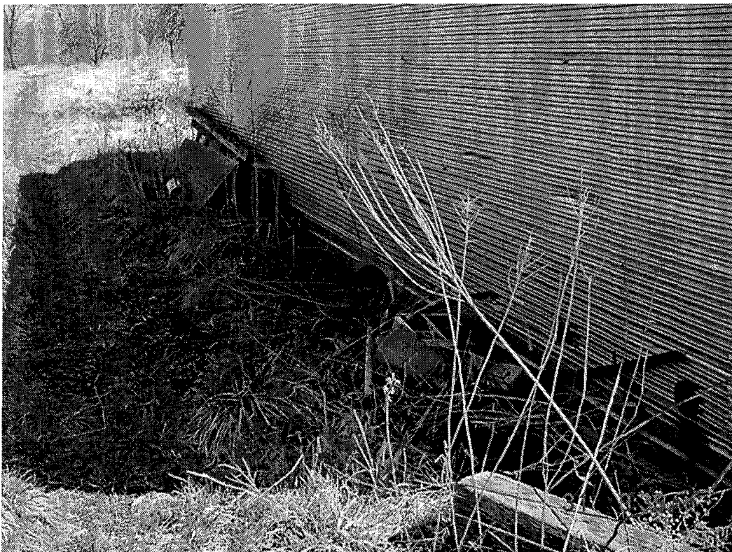
Date: 03/31/2005 Time: 9:39 a.m. Direction: north Photo by: Bill Gonet Exposure #: 008 Comments: Various debris piled along shed.
